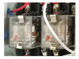
Check whether there is signal output when the time relay is not working.
